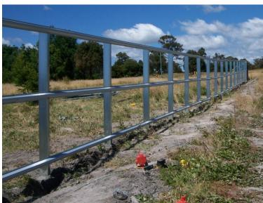
IMPORTANT NOTE: When fixing allow for thermal expansion in the material and do not fix too tightly, each nail should be placed in the centre of the nailing slot and driven in till the head is just clear of the surface of the nailing strip.
