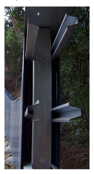
IMPORTANT NOTE: When fixing allow for thermal expansion in the material and do not fix too tightly, each nail should be placed in the centre of the nailing slot and driven in till the head is just clear of the surface of the nailing strip.
