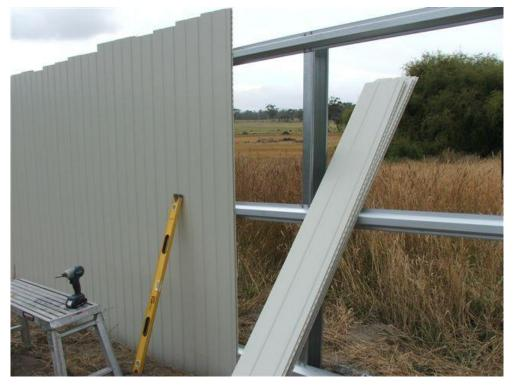
IMPORTANT NOTE: When fixing allow for thermal expansion in the material and do not fix too tightly, each nail should be placed in the centre of the nailing slot and driven in till the head is just clear of the surface of the nailing strip.
